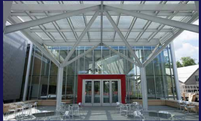
Dickinson College used modern LED fixtures to generate substantial cost savings and sustainability results, while also delivering interior and exterior facility upgrades as well as important safety and security improvements.
