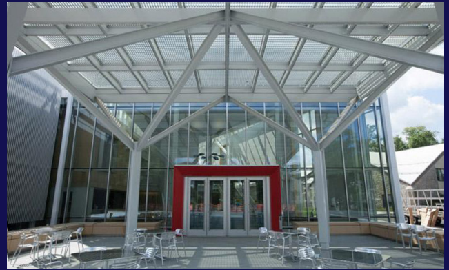
Dickinson College used modern LED fixtures to generate substantial cost savings and sustainability results, while also delivering interior and exterior facility upgrades as well as important safety and security improvements.
